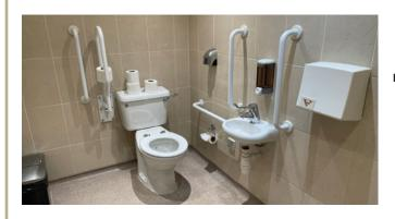
The public accessible toilet is located on the lower ground floor near the restaurant. The accessible toilet feature fixed grab rails and emergency pull cords.
